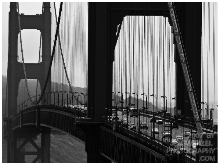
Golden Gate Bridge – San Francisco
